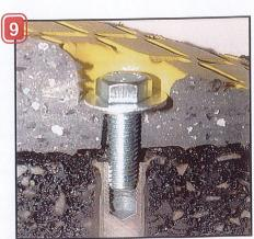
Place the piece to be fixed and tighten with the metal hexagon screw.
