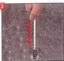
Clean again with a steal cleaning brush and blow off again with a push pump (see picture no.2)
