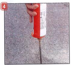
Inject the resin (refer to the fixings indications on the cartridge). Fill the hole by 3/4 We recommend with the use of our resin.
