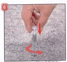
Screw by inserting the ASPHALT FIXING by using the white cap.
