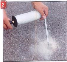
Clean the hole with a push pump. A bad cleaning does considerably reduce the durability and quality of the fixing.
