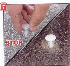
Exact position of the cap during the curing time of the resin.
