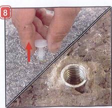
As soon as the resin has hardened, remove the white cap.
